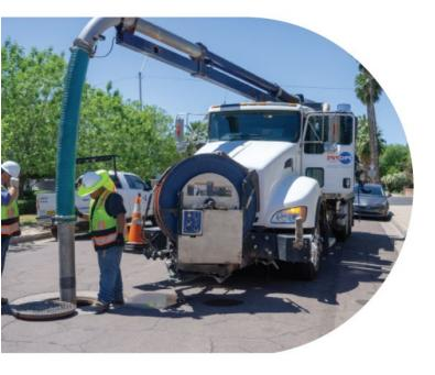
Our customers depend on our industry-leading cleaning capabilities for multiple applications. Cleaning improves the pipe's carrying capacity, recovering its hydraulic efficiency. Extracting debris from the pipe facilitates the insertion and movement of inspection tools through the pipe. Cleaning is often required before undertaking pipe rehab work, such as lining and repairs. Routine cleaning can prevent sanitary sewer overflows (SSOs), which can cause property damage and threaten public health.
